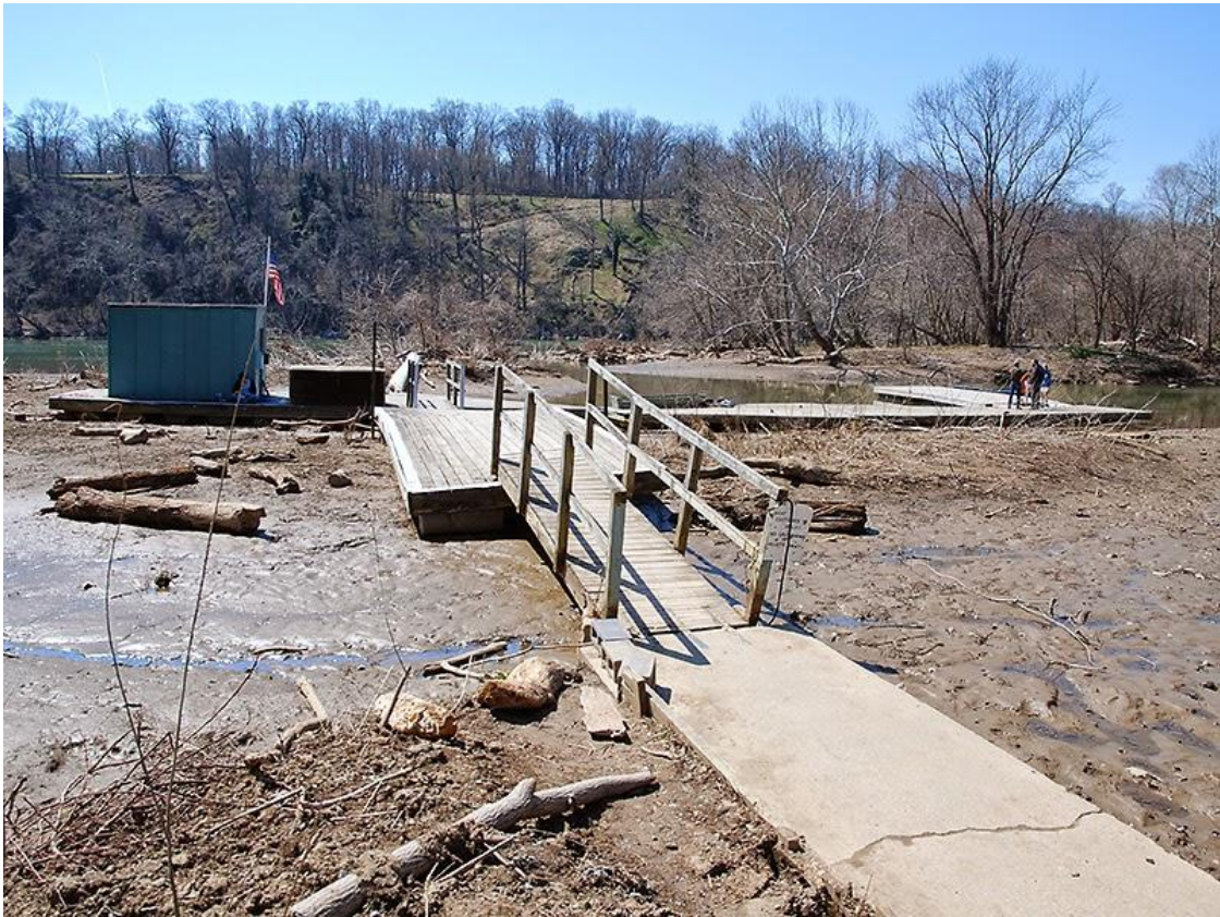
19-20. River Access Closed at Low Tide, 2013 (top); Siltation Around Old Walkway
