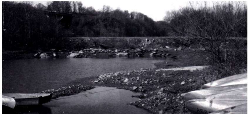
A 1960s construction project altered the natural flow of the river, creating siltation issues at Fletcher's Cove.
